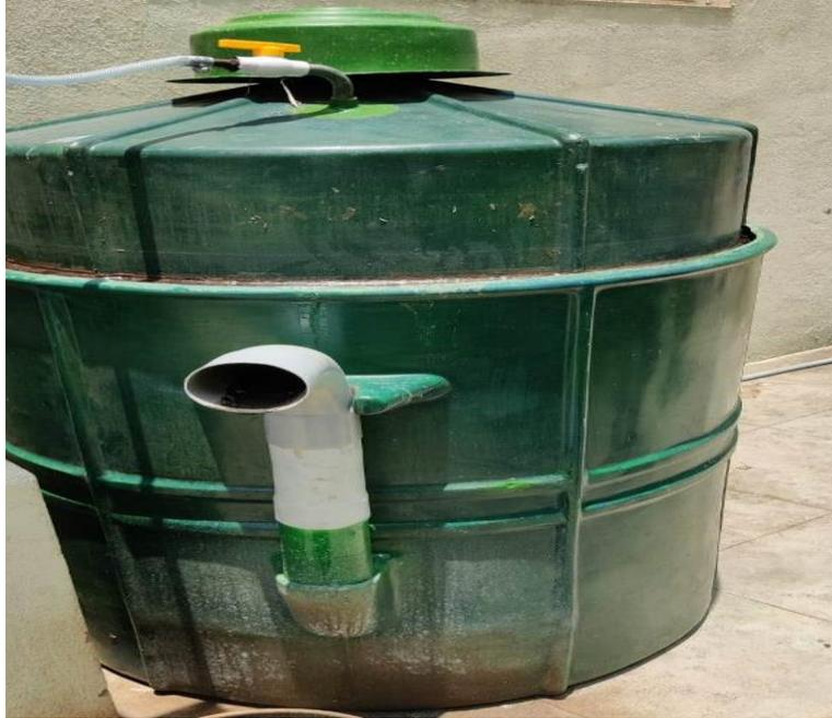
*1m<sup>3</sup> Capacity Bio gas Plant Installed In College Campus*
