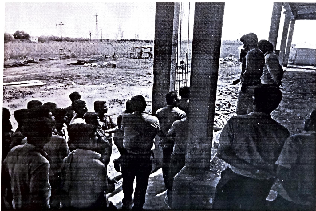
Site Engineer explaining the foundation work followed in agro farm construction
