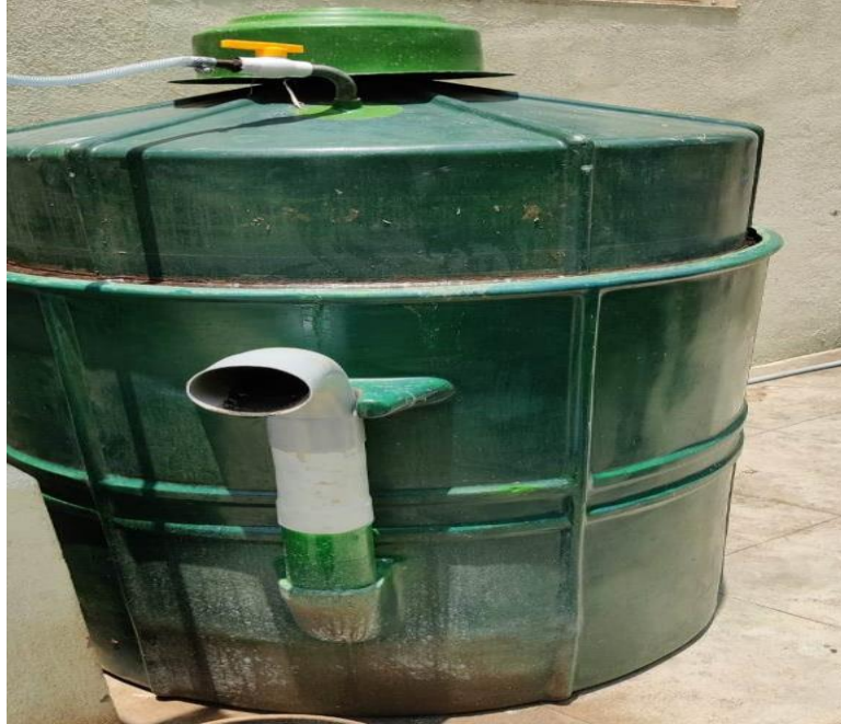
1m 3 Capacity Bio gas Plant Installed In College Campus
